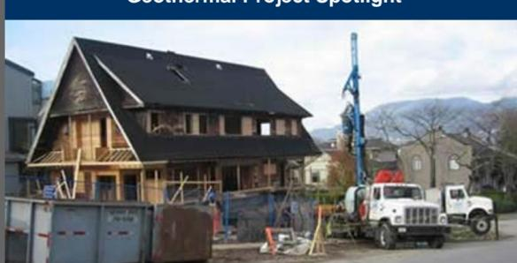
Recently, Sonic Drilling Ltd. was contracted to install four geothermal holes and loops for an older heritage-style home. The home was located on a difficult slope, with tight consolidated material underneath and in the middle of Kitsilano, a popular but congested urban neighbourhood in Vancouver, BC.
