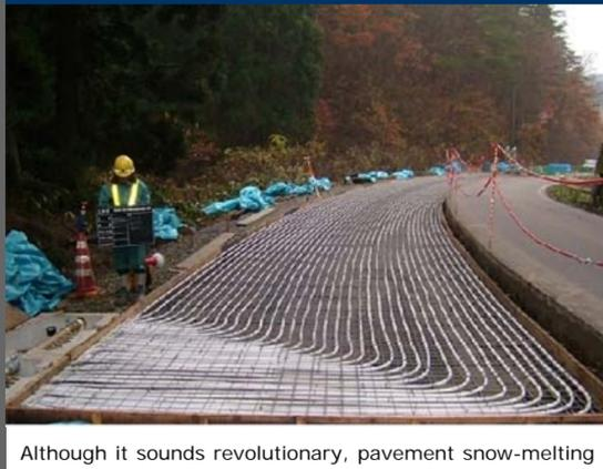
Although it sounds revolutionary, pavement snow-melting technology has been in use in a number of countries including Argentina, Japan, Switzerland and the United States and, in some cases, for as long as 50 years.
