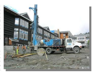
"We are able to complete that many projects as a result of the unique capabilities of the sonic drill, which allows for rapid, simultaneous drilling and casing of the borehole," he says.
