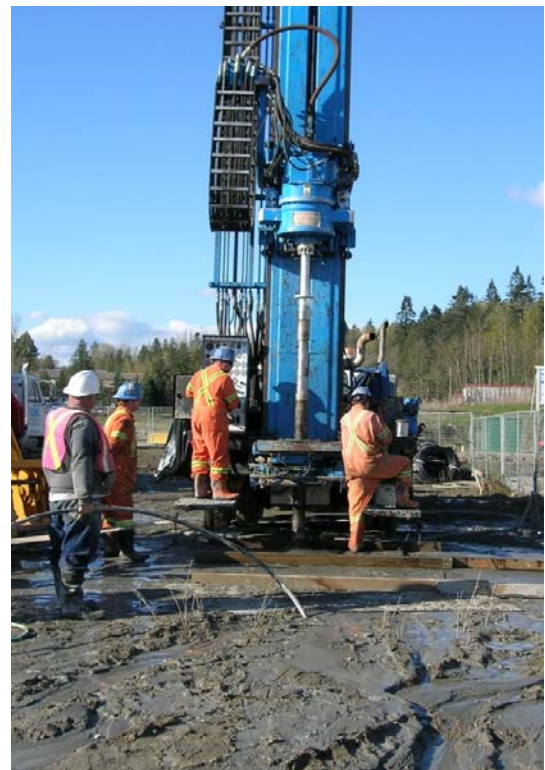
Sonic drill working on site in Langley, BC.
