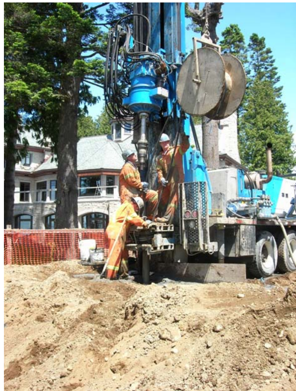
A multi-million dollar home under construction in White Rock, BC, Canada receives a geothermal installation using sonic drilling.
